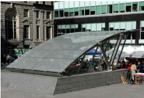
The fritted overhead glass helps reduce solar gain, and distinguishes the canopy’s gracefully curved roof, atop its nearly invisible sidewalls.
