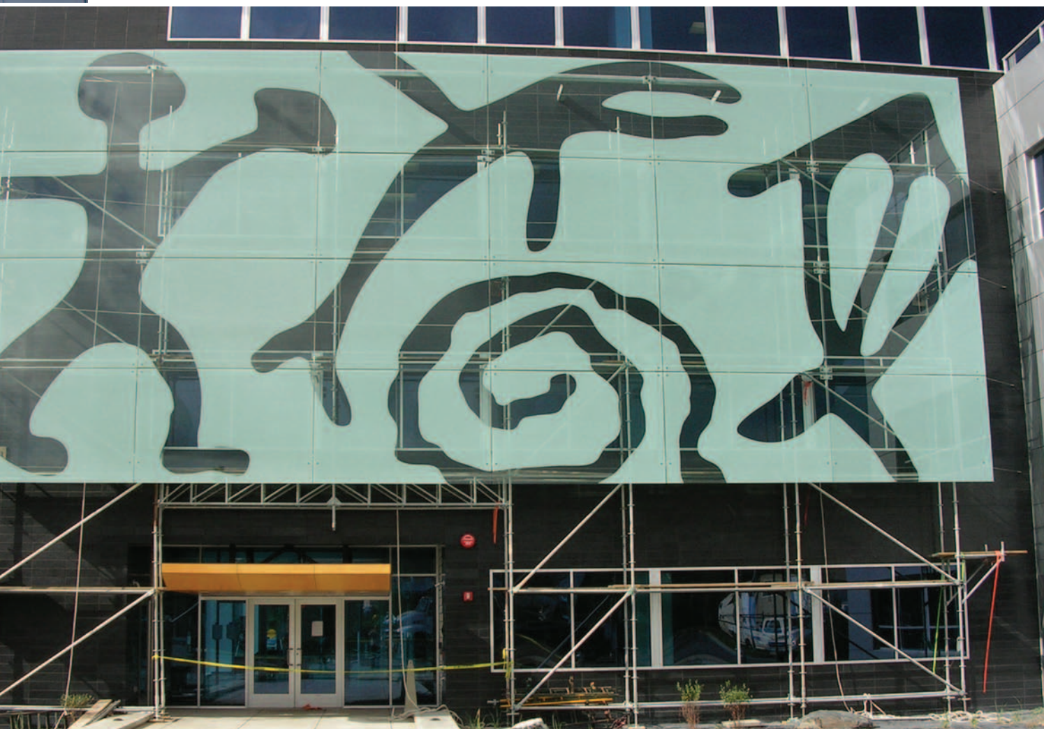
The Afognak project in Alaska features decorative glass screen walls that use the Planar SentryGlas plus system and a simple steel back up.
