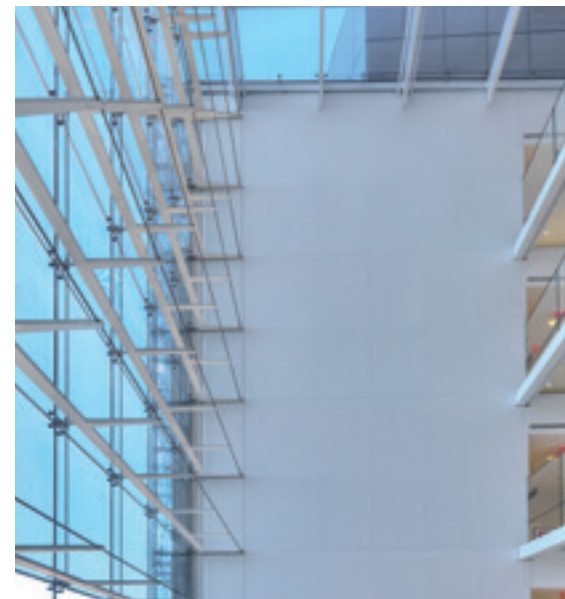
Atrium and entrance enclosures were created using horizontal and vertical tension structures.
