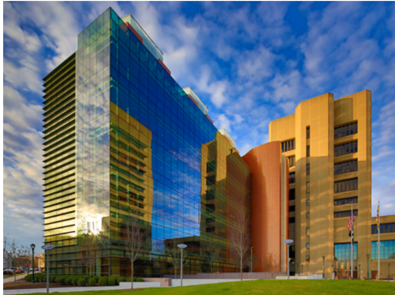
Montgomery County Judicial Center Annex, Rockville, MD, AECOM
