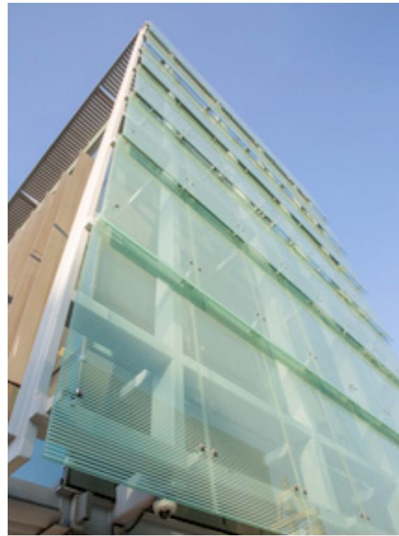
TOP: United Therapeutics Bridge Phase 2B , Silver Spring, MD, EwingCole BOTTOM: Culinary Arts And District Office Building (CAADO) , Riverside, CA, LPA
