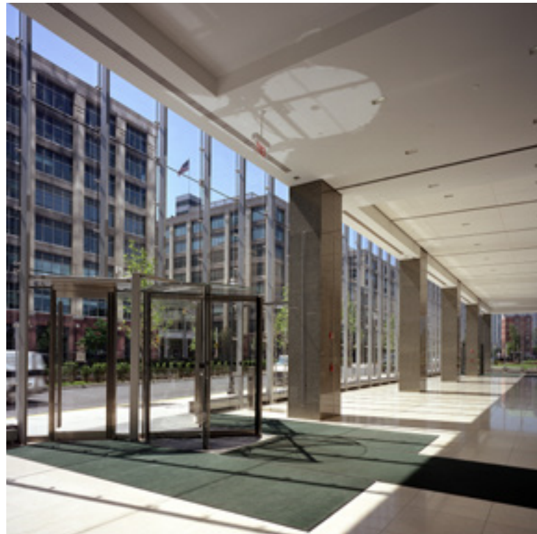
Harborside Financial Center Plaza 5 , Jersey City, NJ, Grad Associates
