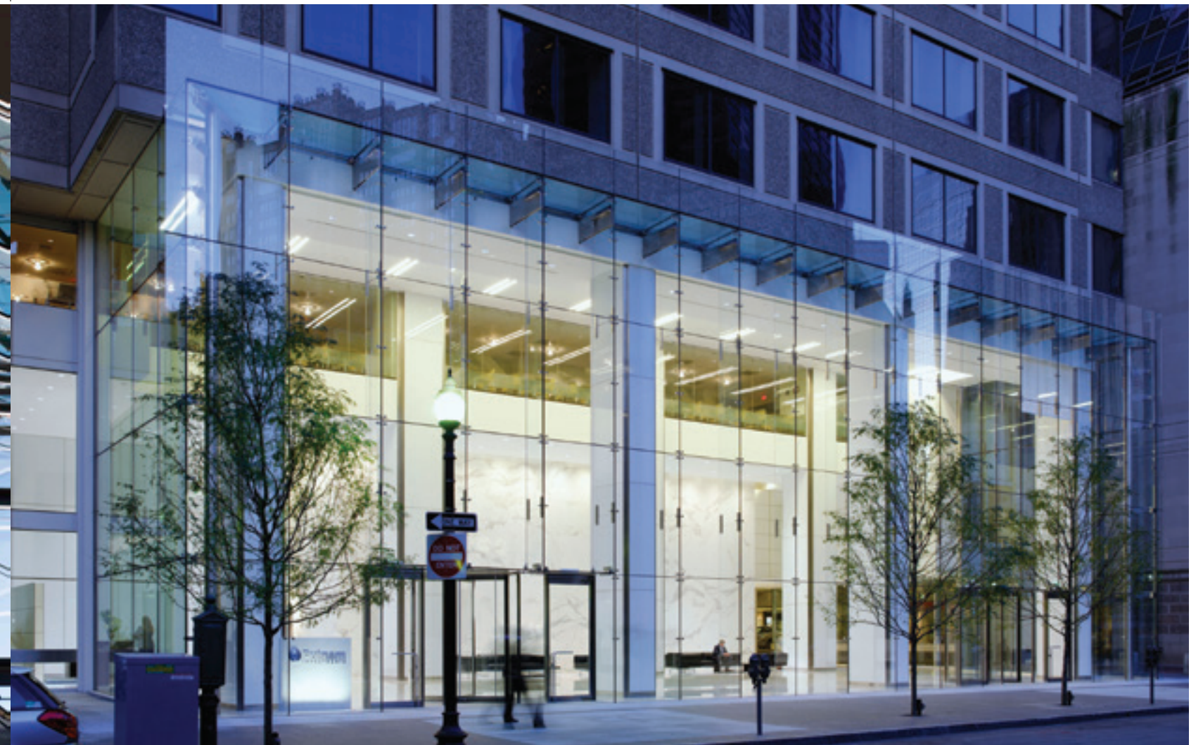
PROJECT One Post Office Square
