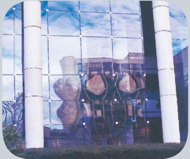
Pilkington **Planar**™ toughened glass exceeds BS EN 12150, ASTM C 1048 and ANSI Z97.1, with maximum optical distortion of 99 milli-diopters (mD) over 95% of the surface for all coated and non-coated glass without ceramic frit, up to 19 mm thickness, while maintaining the minimum stress level required for the Pilkington **Planar**™ system. Mean Roller wave depth 0.02 mm (0.0008") in the central area, for all thermally toughened glass.
